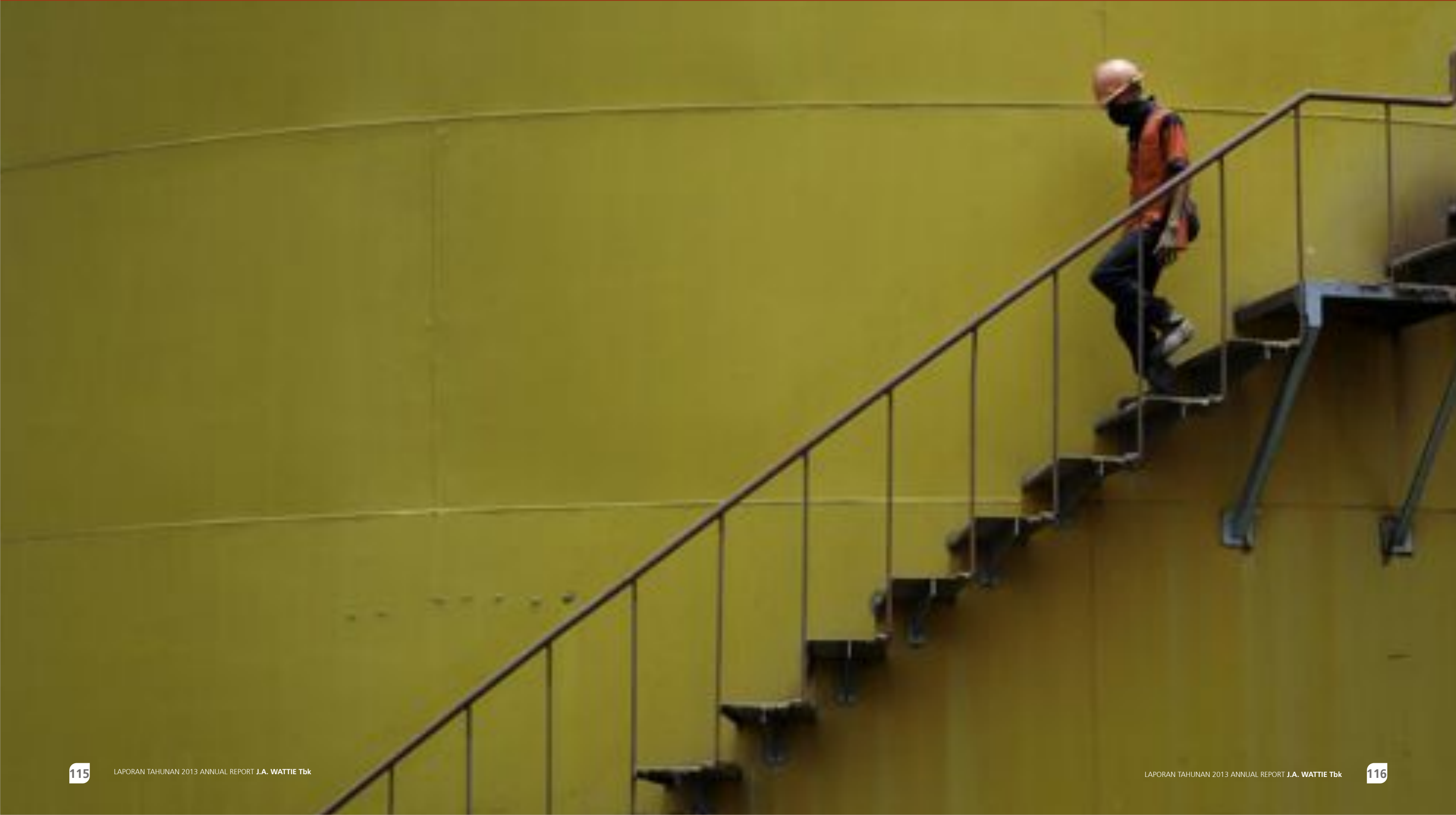
Tangki penyimpanan CPO - PKS Kintap, Kalimantan Selatan. CPO Storage Tank - Palm Oil Mill Kintap, South Kalimantan.
